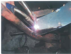
Frame being tack-welded.
