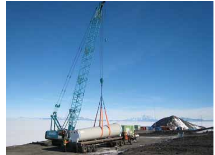
The bottom of the tower section was transported and unloaded ready for assembly at Crater Hill in November 2009. Photo by John Leitch.
