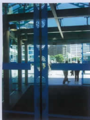
on electronic sliding doors (entrance doors)
