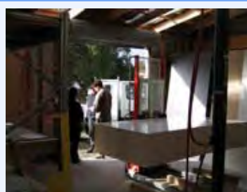
Taking a delivery of boards
