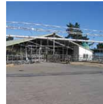
Effluent from 900 cows is collected from a concrete pad waiting area...
